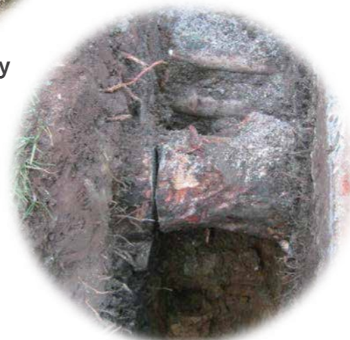
Severely cut / damaged root 根部被嚴重切割或損害
