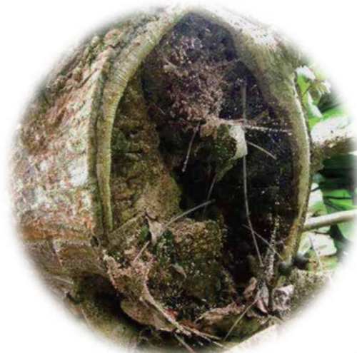
Wood decay / cavity 腐壞 / 樹洞
